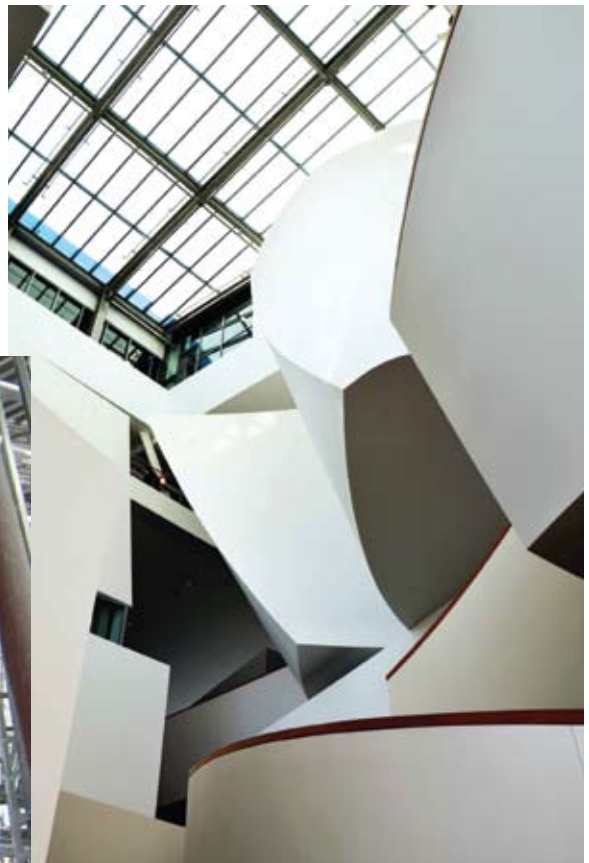
(above) A series of complex curvilinear shapes comprise the interior of the New World Symphony's Campus Expansion in Miami. Framing was rendered in 3D by Radius Track, using data from architect Frank Gehry's computer-based designs.
