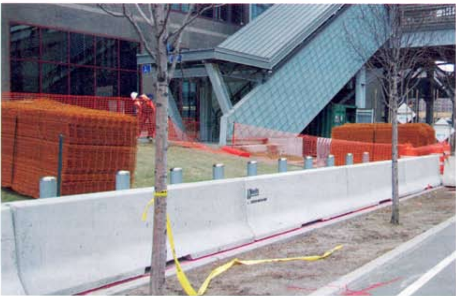
Barriers protect WTC transportation hub.
